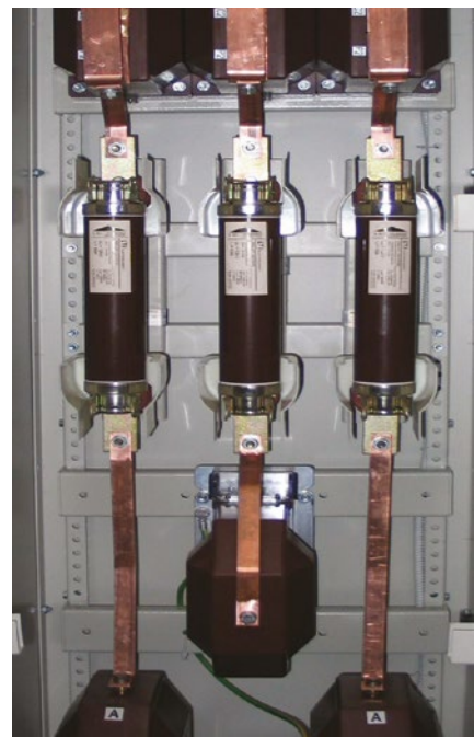
Connection in indoor switchgear, example:
